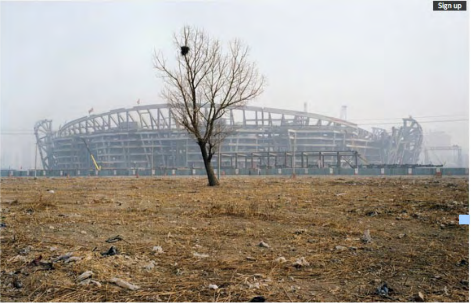
† Top: June, 1994. Above: Olympic Stadium, 2005-2008
