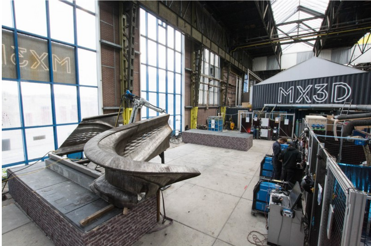
A look inside of the factory producing the world's first 3-D-printed bridge. Photo: Courtesy of MX3D
