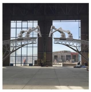
The versatile six-axis <u>robots</u> – which are able to rotate their arms along six different planes of movement – will print a loadbearing structure that will support their own weight as they work.
